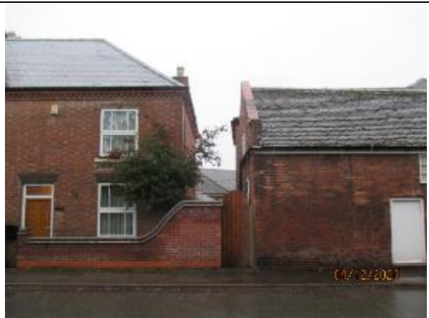
Gap between 259 and the adjacent home, site of the proposed link building
